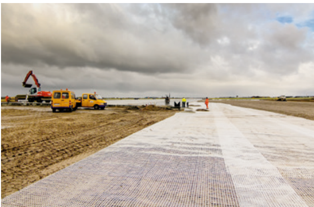
Figure 5 Large-scale installation of a Secugrid® reinforced base course
