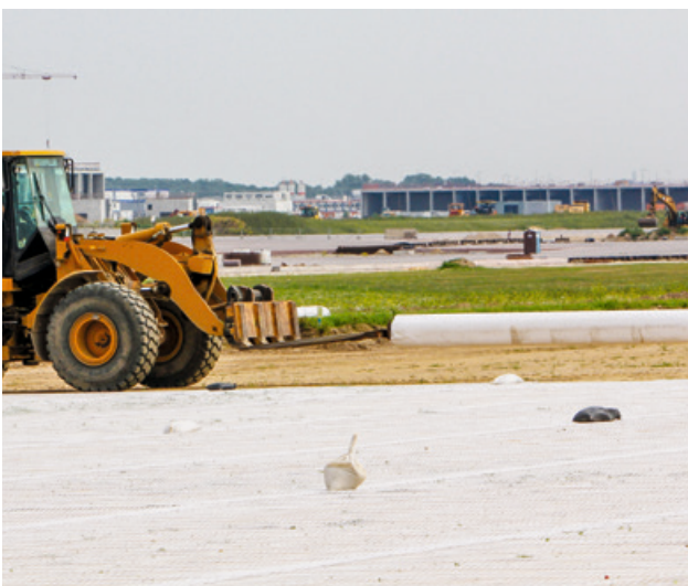
Figure 11 Installation of Secugrid® (no pre- stressing required)
