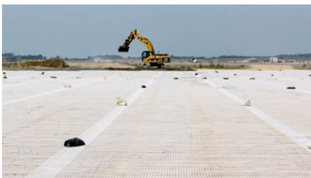
Figure 7 Installation of base course aggregate on top of Secugrid®
