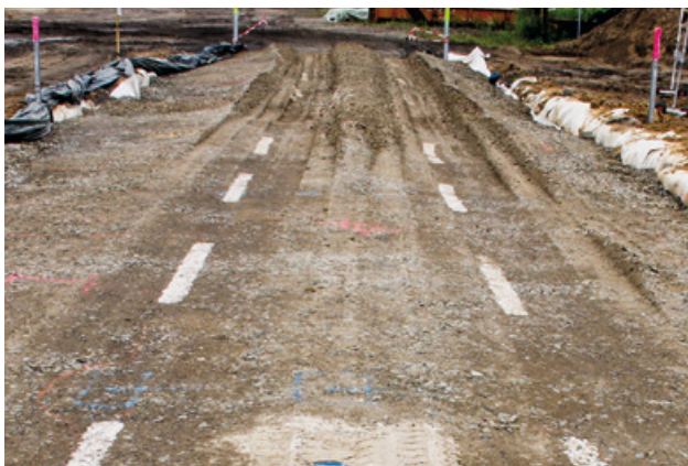
Figure 21 Low rut depth in the Secugrid® geogrid reinforced test section (in the front) compared to the unreinforced test section (in the back)
